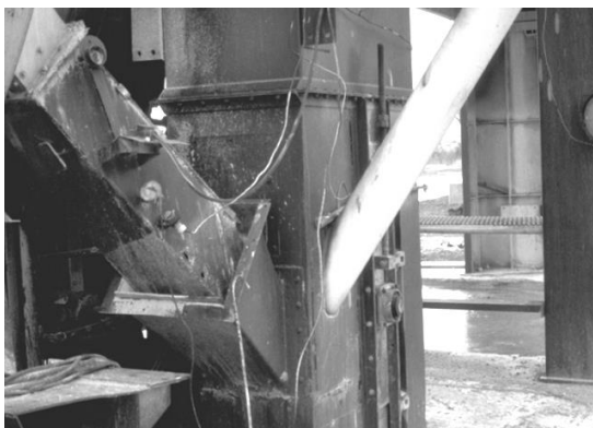
Base of the Hot Elevator
