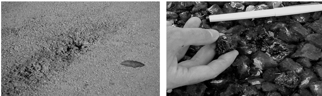
Effects of Liquid Asphalt Binder Stripping
