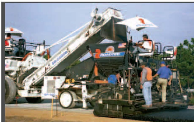
SHUTTLE BUGGY MATERIAL TRANSFER VEHICLE BY GRAVITY AUGER F37
